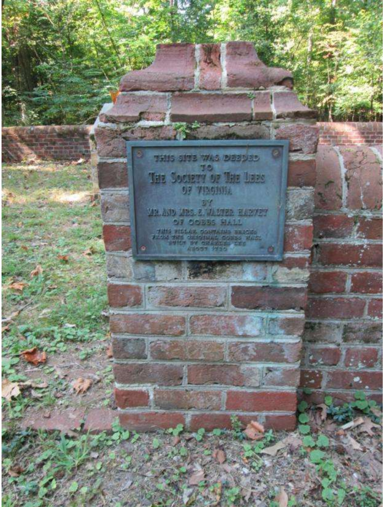
Right Entrance Pillar, September 12, 2013
